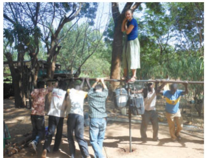
Well-drilling in Burkina Faso an example of teamwork. Lindsey Adomat '14 helps stabilize the human-powered drill.
