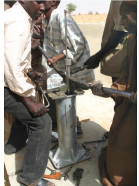
*Well technicians installing a hand pump in Niger.*
